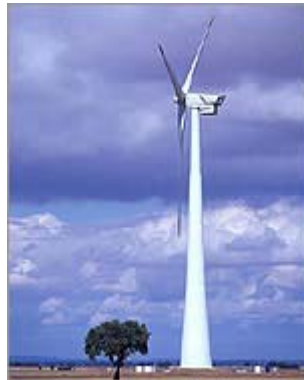
GE Wind Energy's 3.6 megawatt wind turbine is one of the largest prototypes ever erected. Larger wind turbines are more efficient and cost effective.
